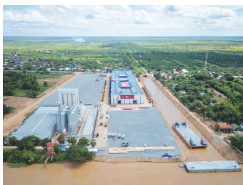
Techo Funan Canal
